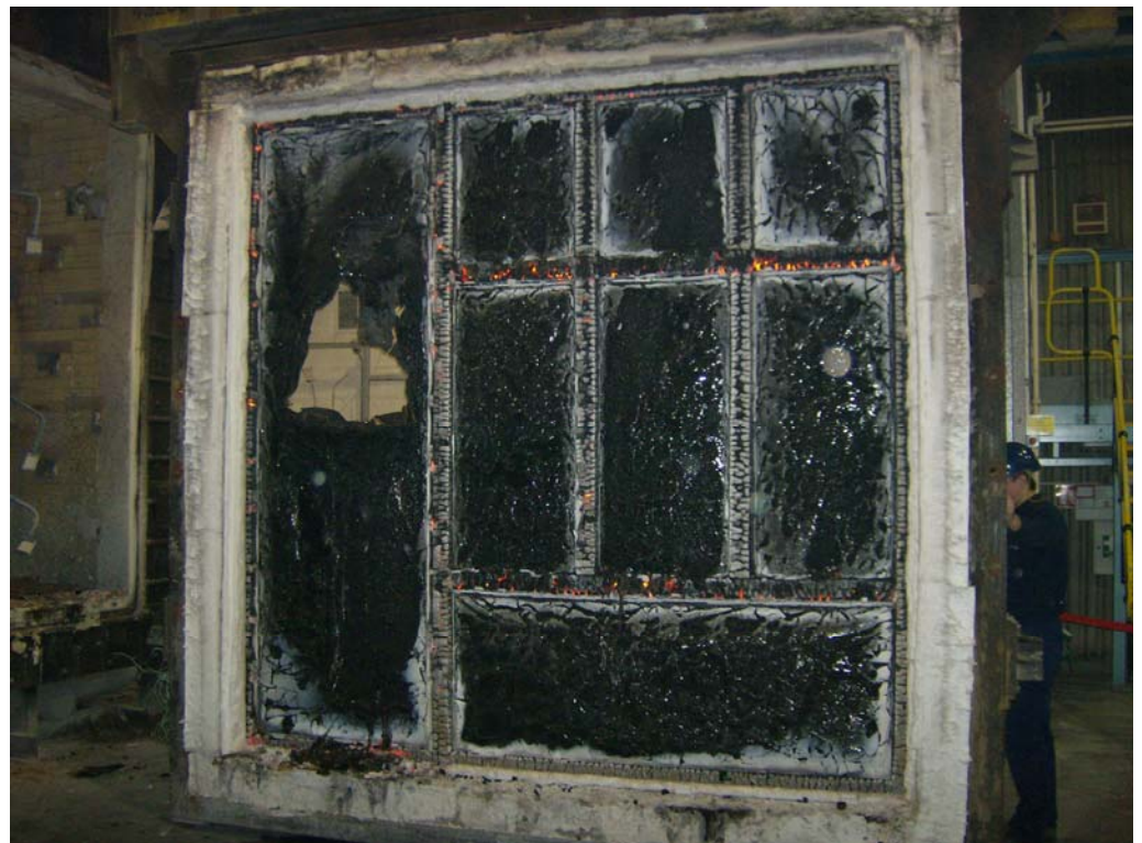
The exposed face of the test construction directly after the test
